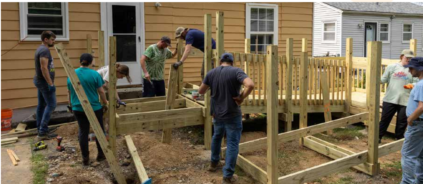
Building a new wheelchair ramp
