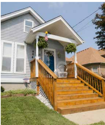
New entry stairs
